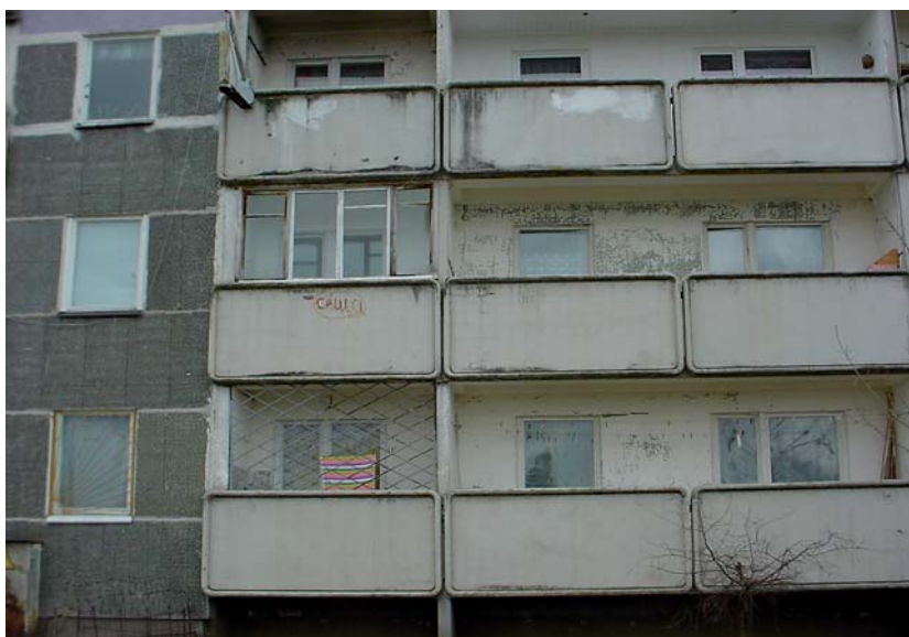
Detail of a system-built residential building in Jelgava, 2003
