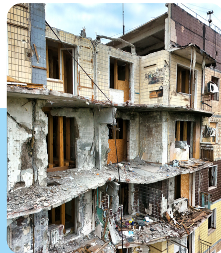
Rehabilitation of a multi-storey building in Kryvyi Rih after a missile attack
